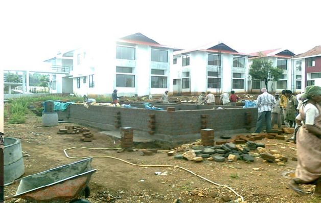
Starting of construction of Cottages under Phase 3
