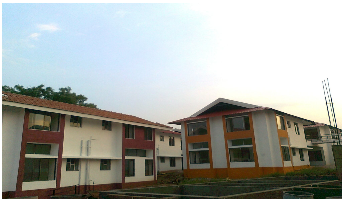
Some of the Cottages in Phase 2 ready for occupation
